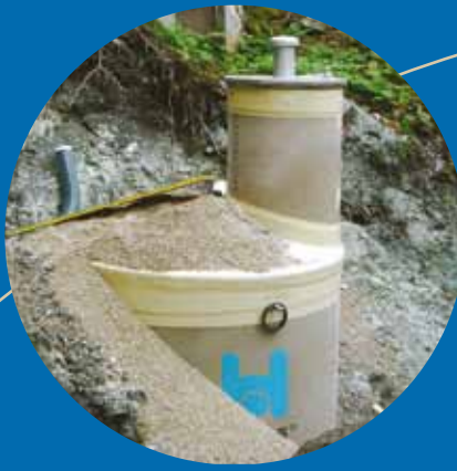
Spring water collection shaft
