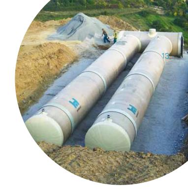
units as well as the broad range of fittings such as bends, tees, y-junctions, etc. either consist of pipes segments, which are assembled and firmly joined with laminate or they are fabricated by wet molding, SMC (Sheet Molding Compound) pressing to fiber spray lay-up.
