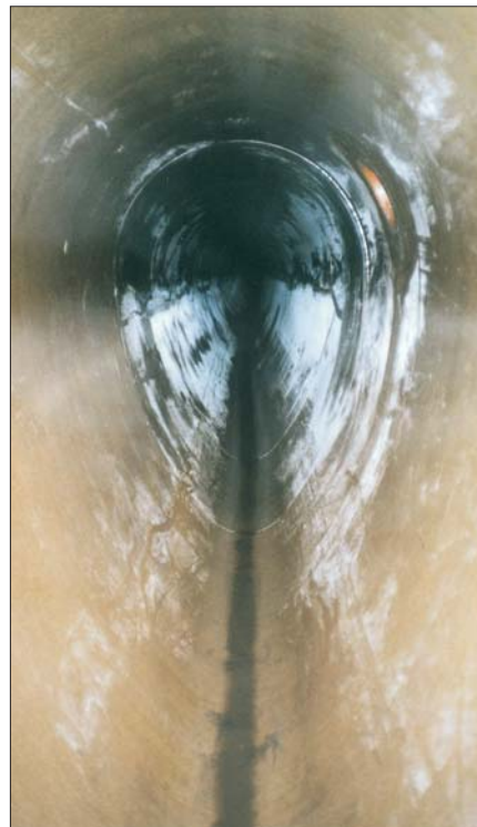
Rehabilitated sewer with DN 200 laminated inlet
