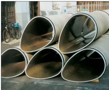
HOBAS NC Line Products DN 680/1050 for Relining stored in front of the access shaft
