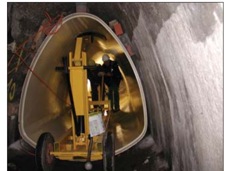
HOBAS NC Line pipe installation
