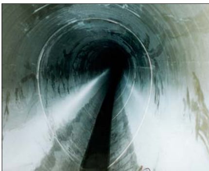
View into the rehabilitated sewer
